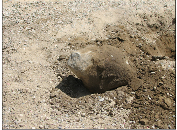
The stone removed from the road.
