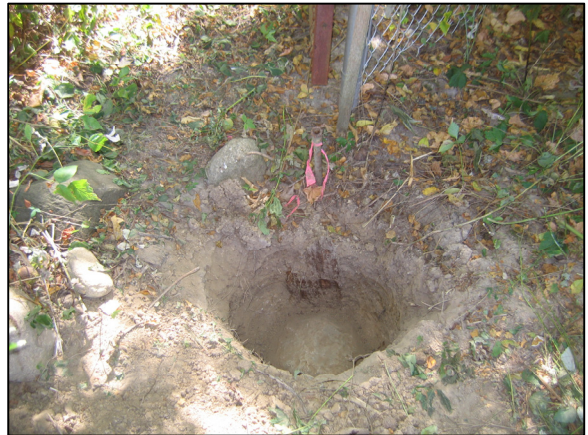
Corner 2 being excavated, showing the pipe, metal posts to the south, the in ground portion of the wood post, and a rock found on the north side of the post, presumably a brace rock.
