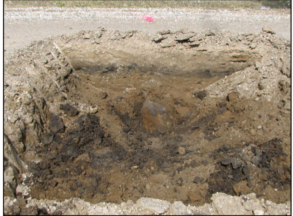
View of the stone and cross section of the road from the south.
