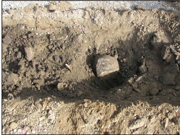
View of the stone and rebar.
