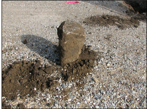
The stone removed from the road bed.
