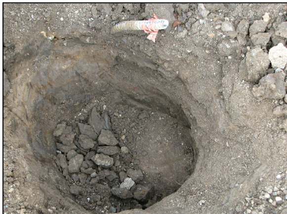
View of the lower stone and rebar.
