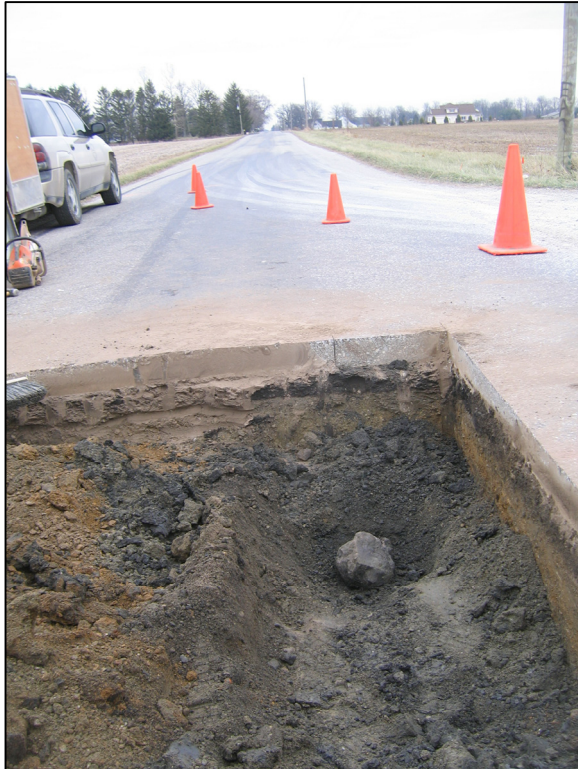
View of the stone and County Road 100 North, from the west, looking east.
