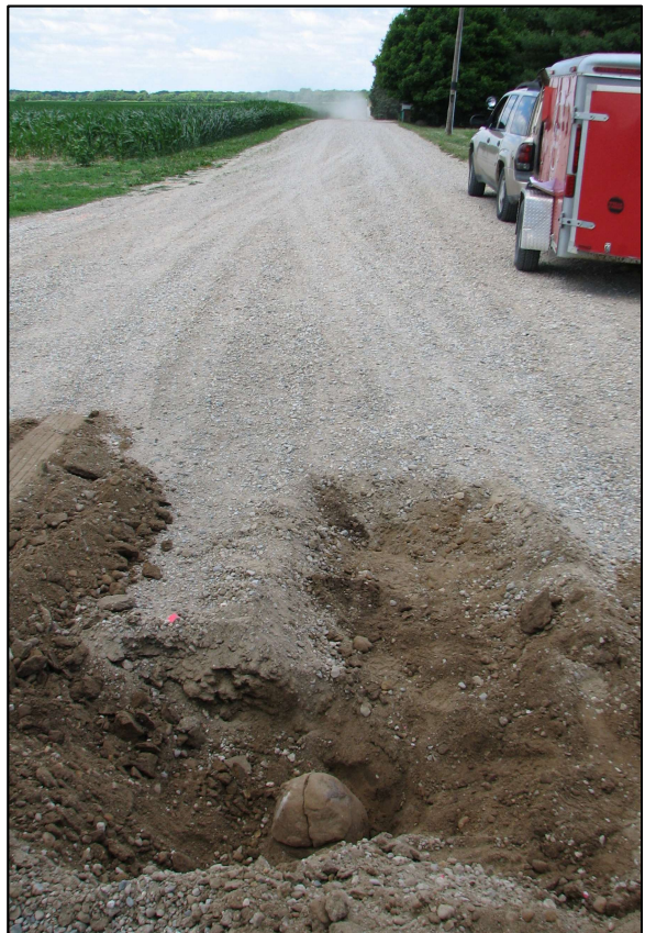
View from the east, looking across the stone and west along C.R. 750 North.
