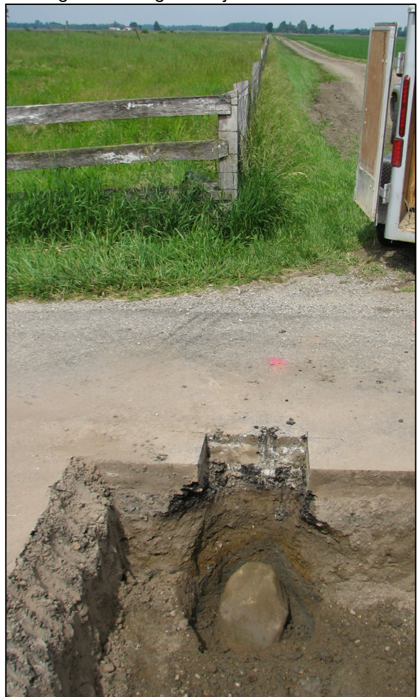
View from the east, looking west along the adjacent fence line.
