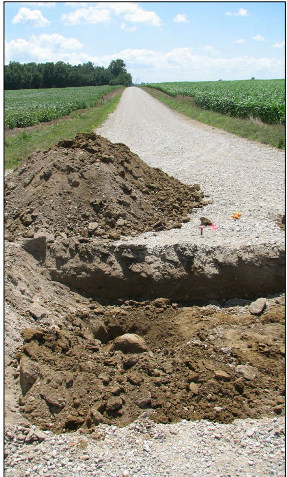
View from above the stone, looking South along County Road 800 East.
