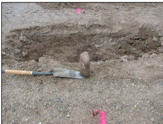
The stone removed from the road.
