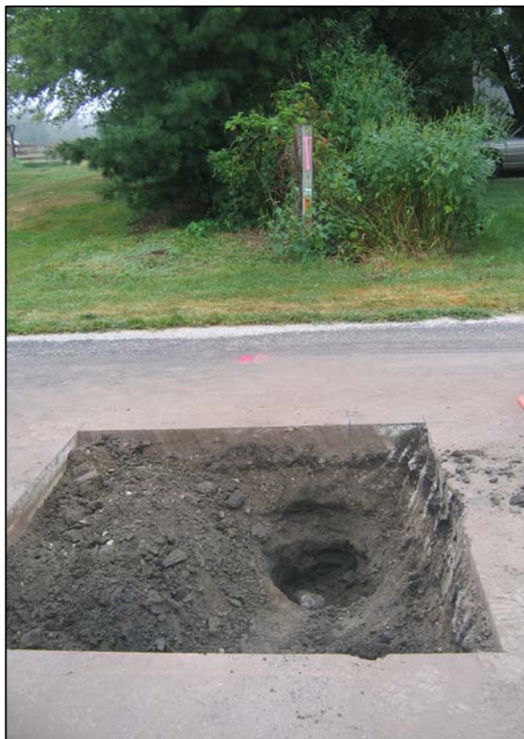
View from the north, looking across the lower stone towards the post and trees to the south.
