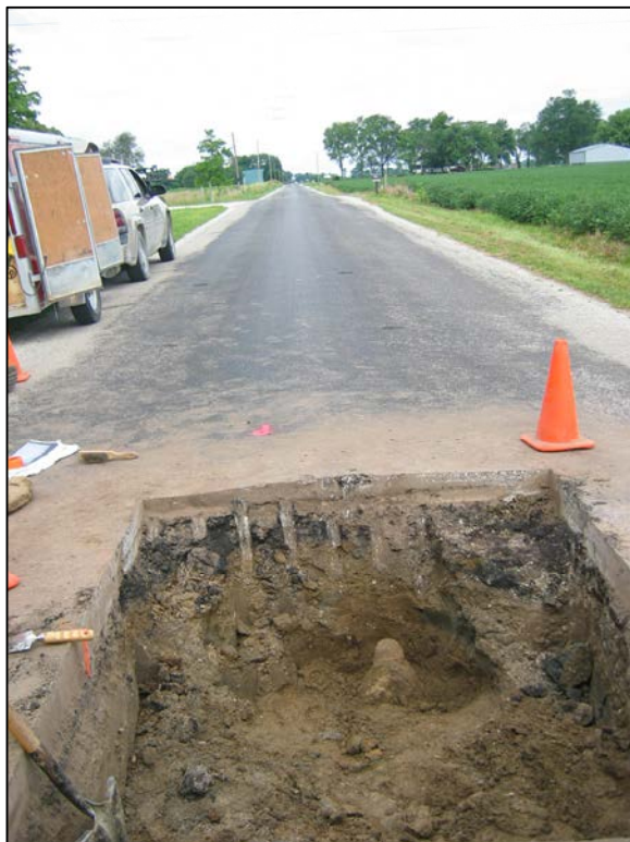
View of the top record stone and brace rock from the east, looking west along C.R. 100 North.
