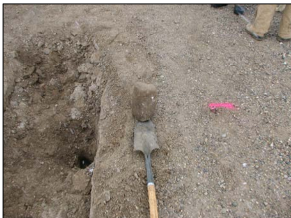
The stone removed from the road.
