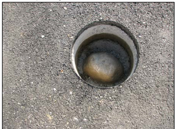
View of the stone from above, immediately prior to the top being encased in concrete.
