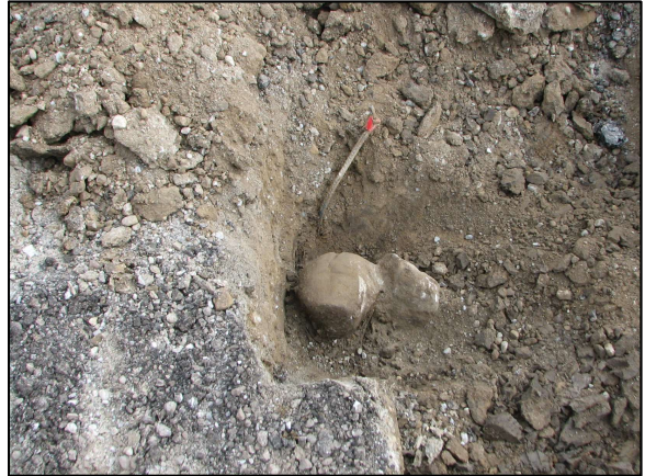
Both stones and the rebar.
