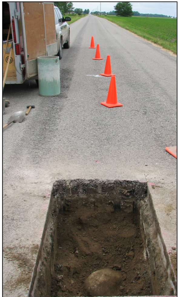
View of the stone as it is situated in within County Road 200 North.
