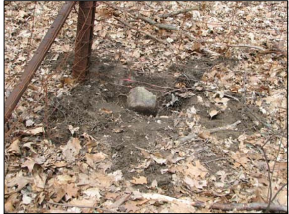
Corner stone with some of the stone exposed - overhead view from southeast.
