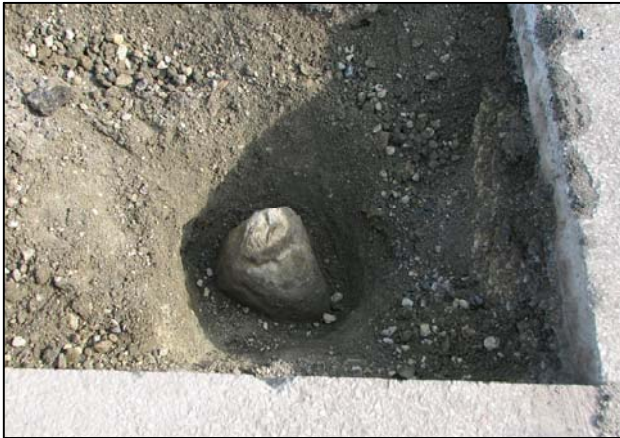
Corner stone - overhead view from south.
