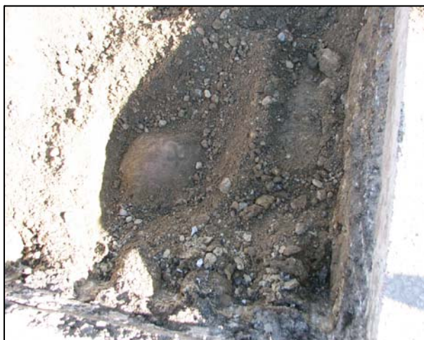
Corner stone - top exposed.
