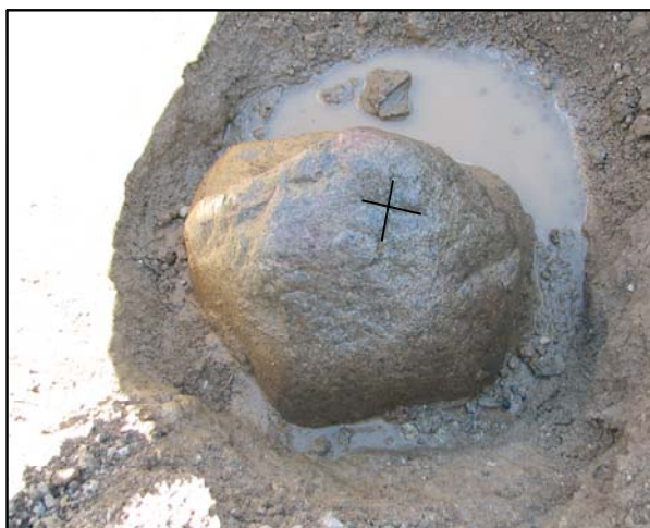
Corner stone - close up with etched "+" enhanced for ease of visual detection.
