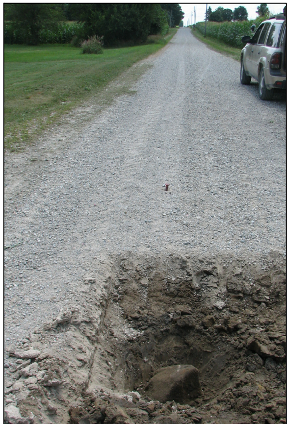
View from the north, looking across the stone and south along County Road 800 East.
