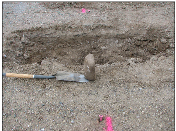
The stone removed from the road.
