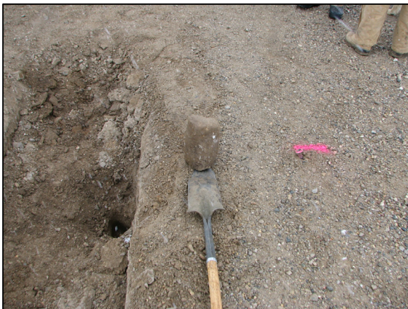
The stone removed from the road.
