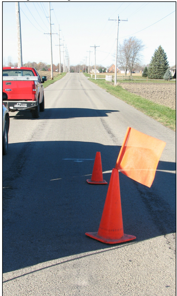
View from over the stone, looking west along C.R. 300 North.
