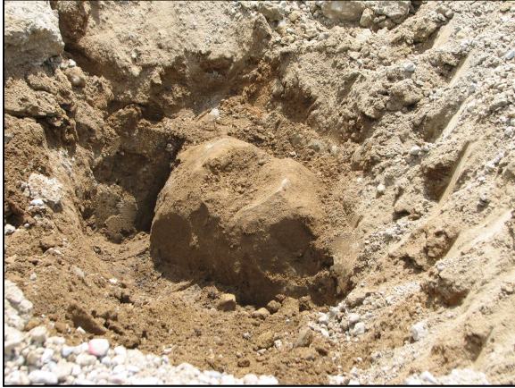
The stone partially exposed, view from above and north.
