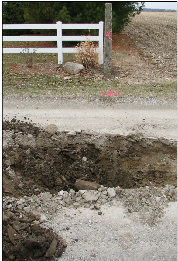
View from the east showing the stone and the post on the west side of the road.
