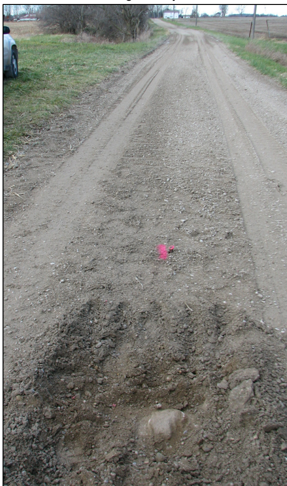
View from the south looking across the stone and rebar and north along County Road 900 East.
