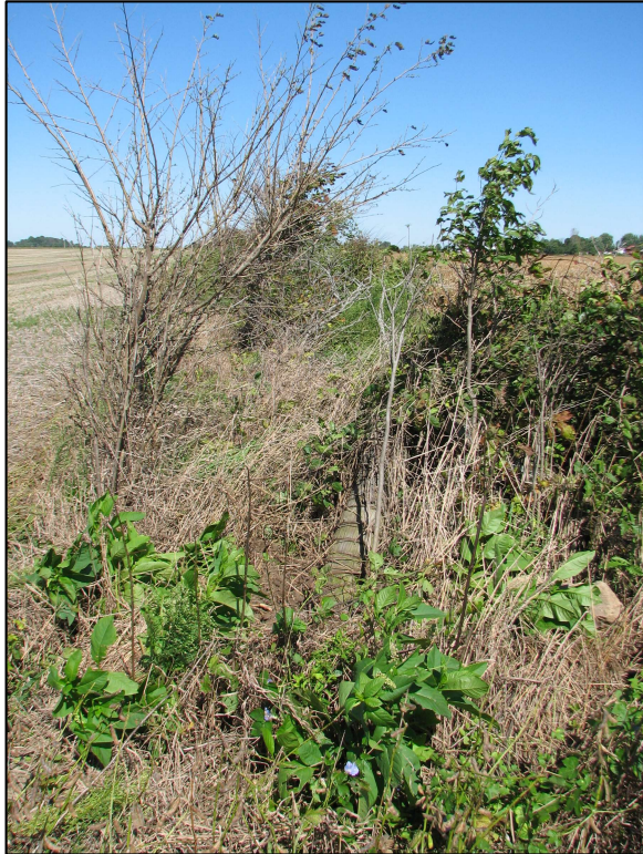
The corner prior to excavation. View of the leaning corner post from the south.
