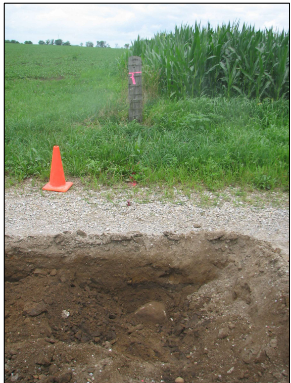
View of the stone and the post on the north side of County Road 900 North.
