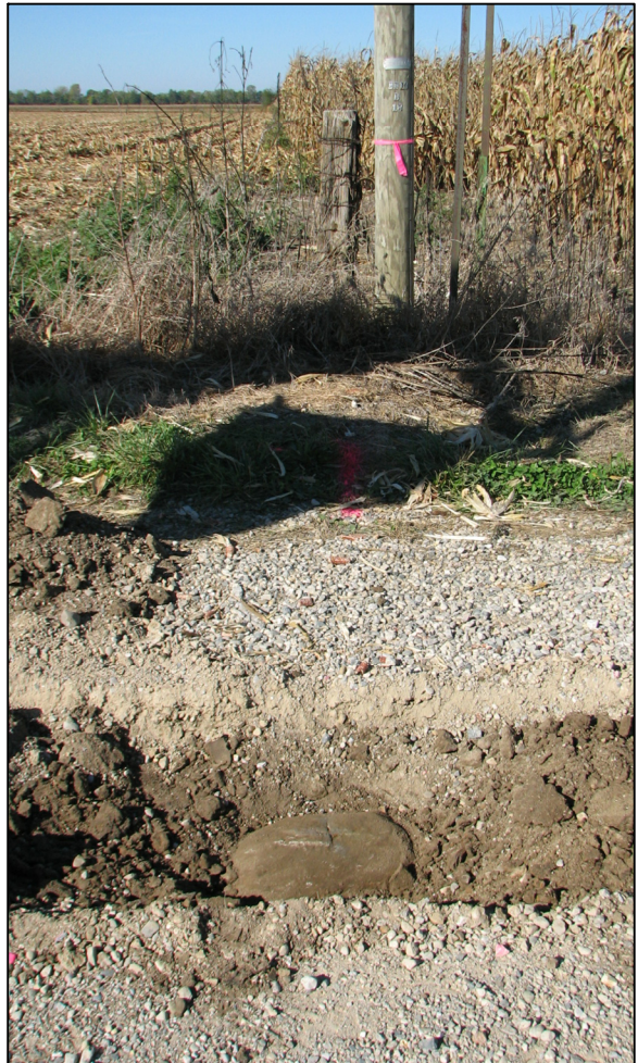
View from the east, showing the stone and the old end post on the west side of the road.
