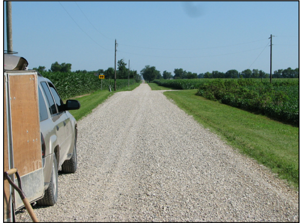
View prior to excavation, looking north along Meridian Road from above the closing corner.
