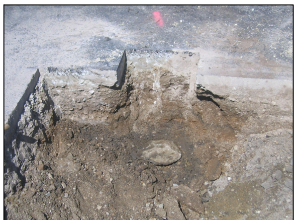
The stone at the standard corner (corner 1) from above and east.
