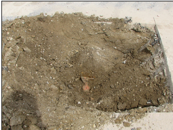
View of the top of the railroad rail as found.
