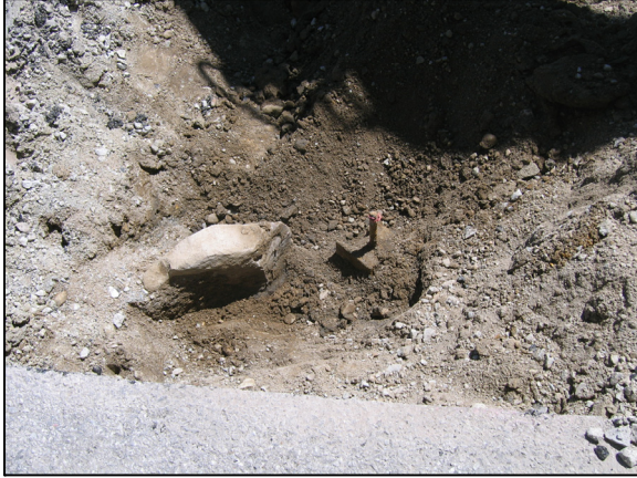
The first stone found with the rebar and railroad rail.
