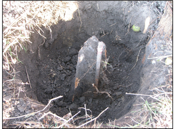
The base of the old post, with rebar.
