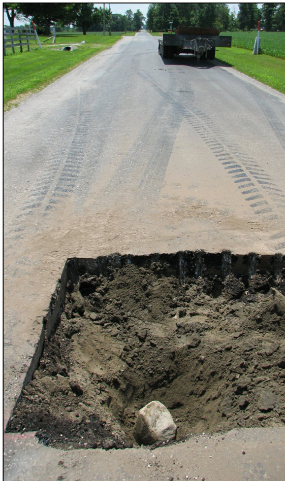
View from the north, looking across the upper stone and south along County Road 500 East.
