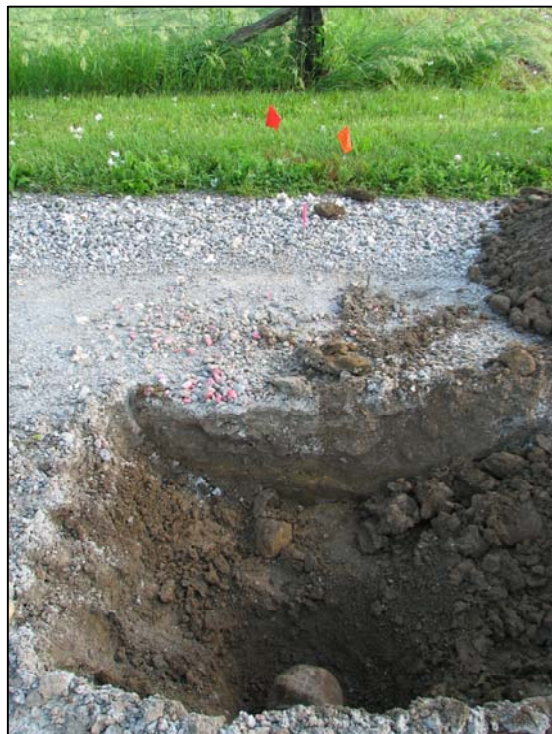
View from South looking over stone to wood corner post.
