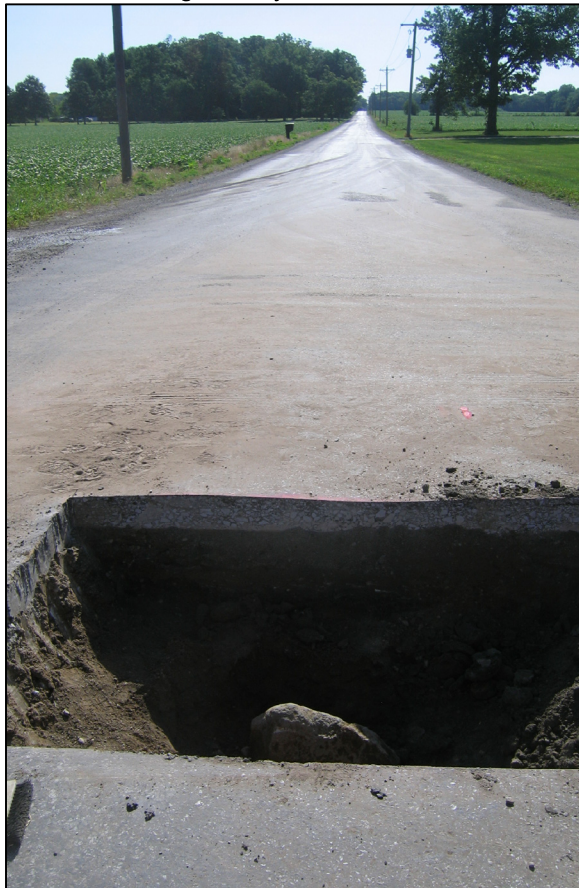
View from the west, looking across the stone and west along County Road 100 South.
