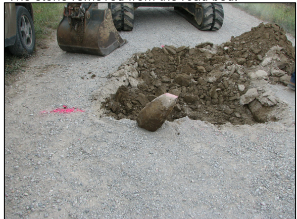
The stone removed from the road bed.
