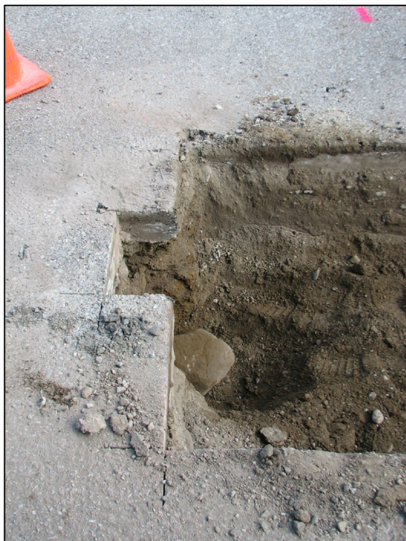
View of the stone from the south.
