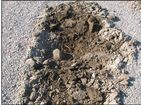
The stone and rebar as originally exposed.
