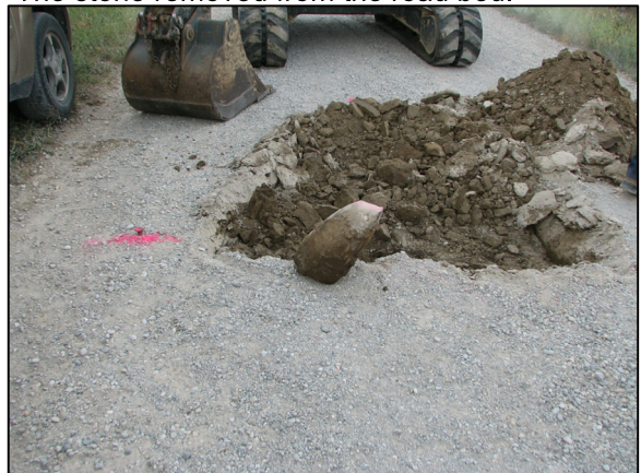
The stone removed from the road bed.
