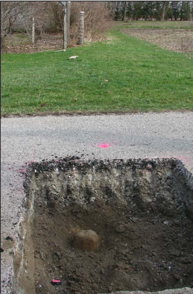
Corner stone - view from South.
