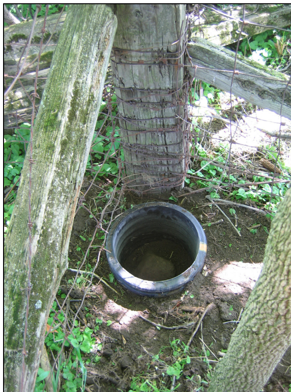
A vertical section of plastic storm pipe set around the stone. The stone was left as found, but surrounded by the section of storm pipe.
