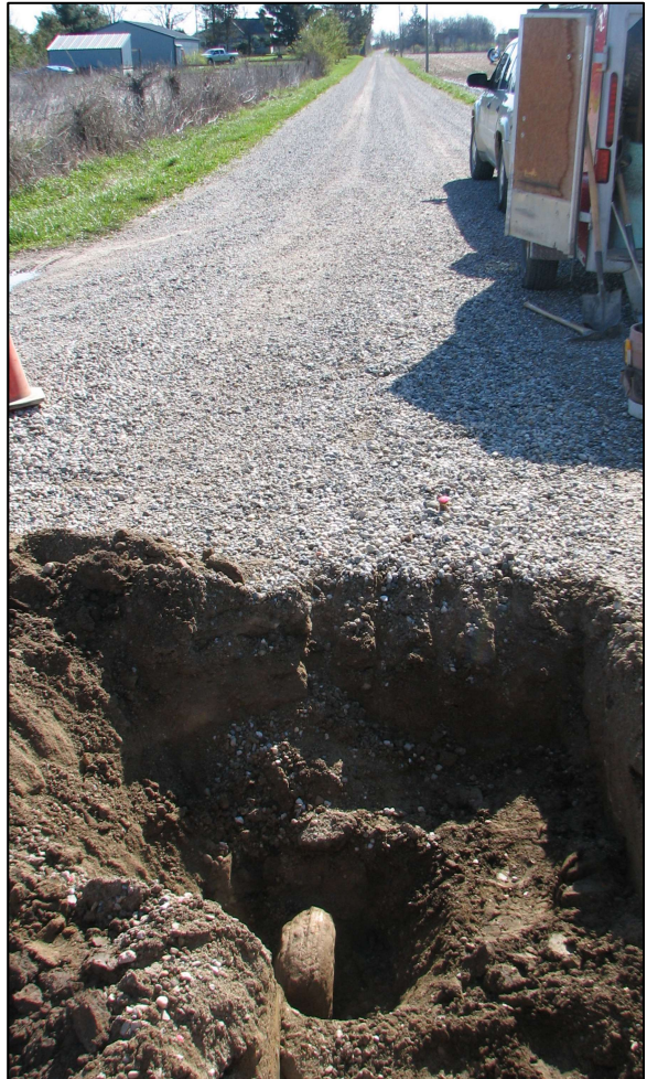
View from the west, looking across the stone and east along County Road 150 South.
