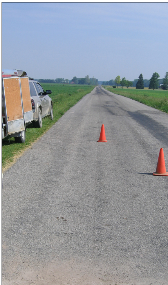
View from above corner 2, looking north along County Road 600 East.
