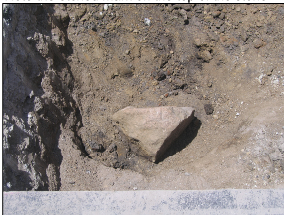
The stone at corner 2 from above. Note the etched mark on the top of the stone.
