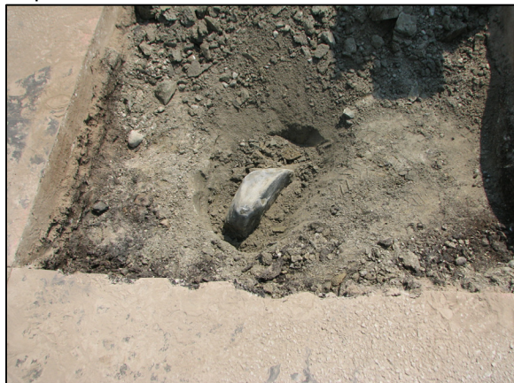
The stone at the stanard corner more fully exposed. View from above and west.
