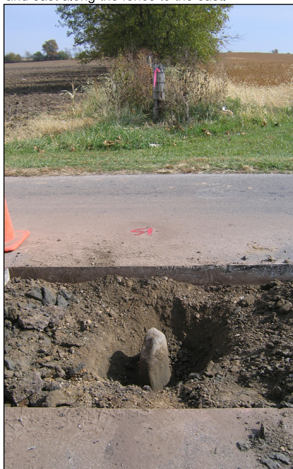
View from the west, looking across the stone and east along the fence to the east.
