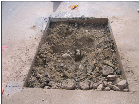
View of the stone as first exposed, along with the railroad rail.
