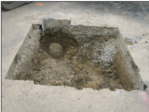
The stone and area of excavation from the east.
