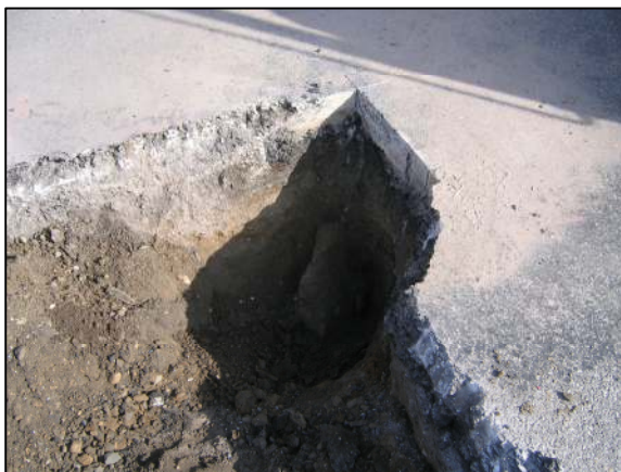
Similar view to above. View from the southwest.
