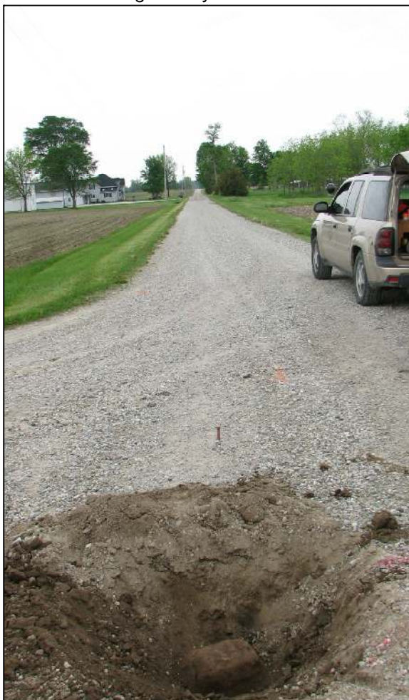
View from the north looking across the stone and south along County Road 300 East.
