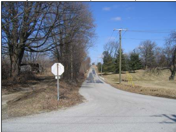
View from standing upon the harrison monument / stone, looking north along County Road 800 East (Kissel Road).
