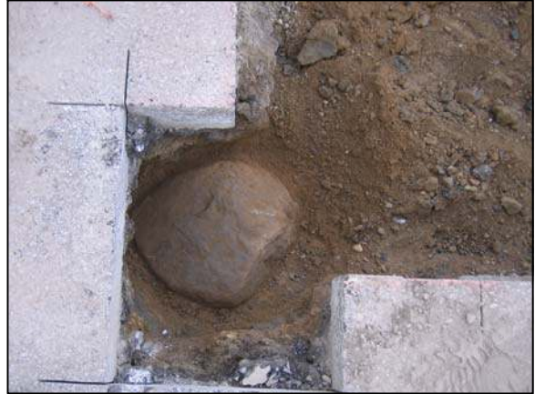
Corner stone. View from above.
