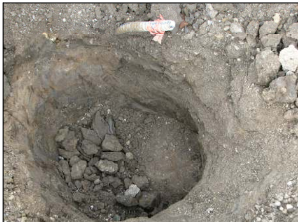
View of the lower stone and rebar.
