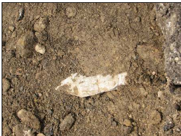
The top of the stone from above after fill material was packed back around the stone.
