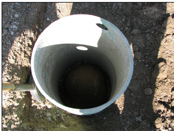
The stone before the top was encased in concrete and the harrison monument set.
