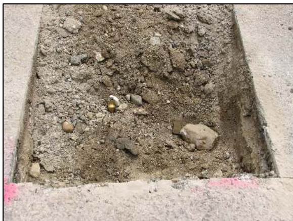
View from above and north, showing the stone and the position of the rebar as marked with a plumb-bob.
