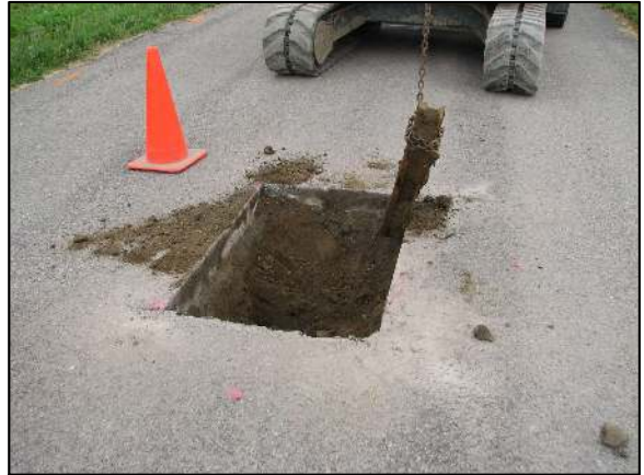
The railroad rail being removed from the hole.
