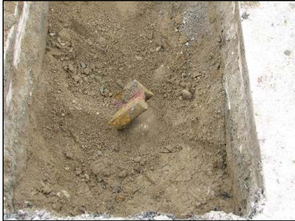
The top of the railroad rail found leaning over the stone.
