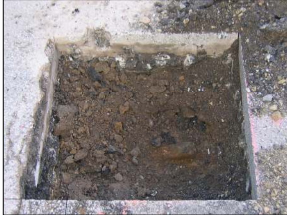
View of the railroad rail as first exposed.
