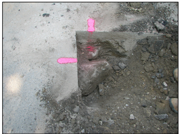
The various found stones and the area of excavation prior to patching the road bed.
