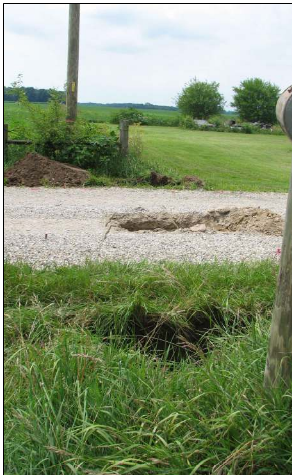
View from NNE, showing the three areas of excavation (see Section Corner Record).
