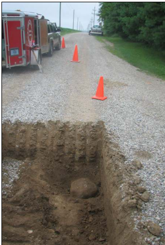
View from north, looking across the stone and south along C.R. 1100 West to the south.
