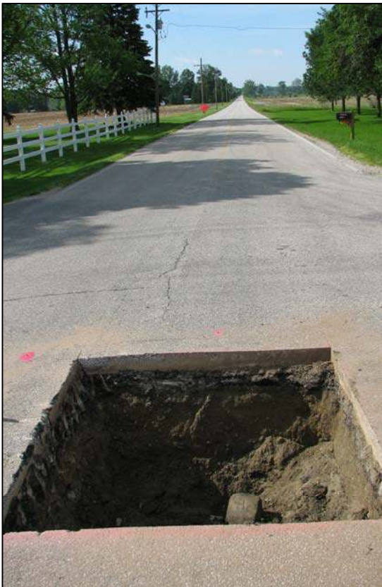
View from South showing County Road 650 East to the North.
