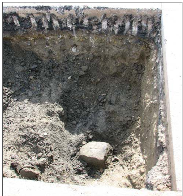
Overhead view from West.
