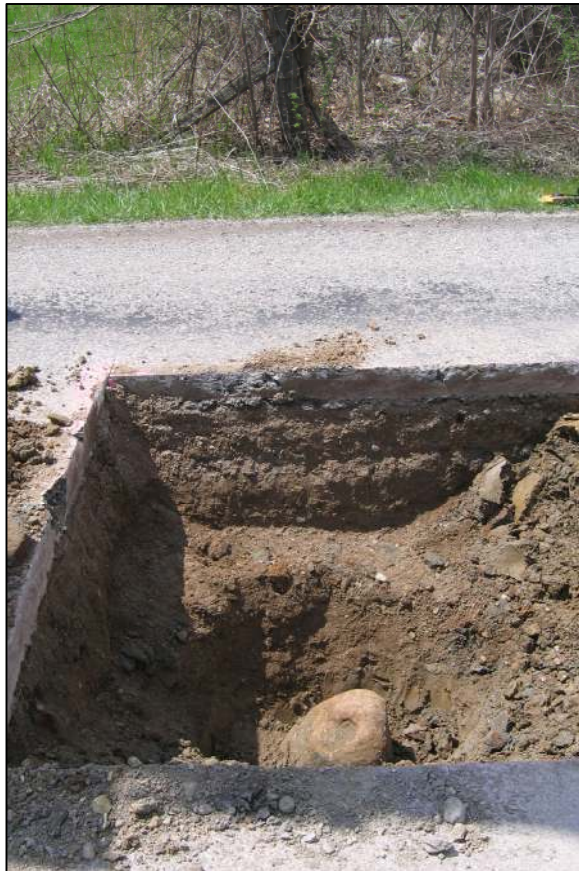
View of the stone and the wood end post on the east side of the road.
