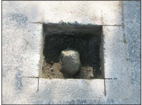
View of the stone as exposed on 5/11/2011, immediately prior to being encased in concrete.
