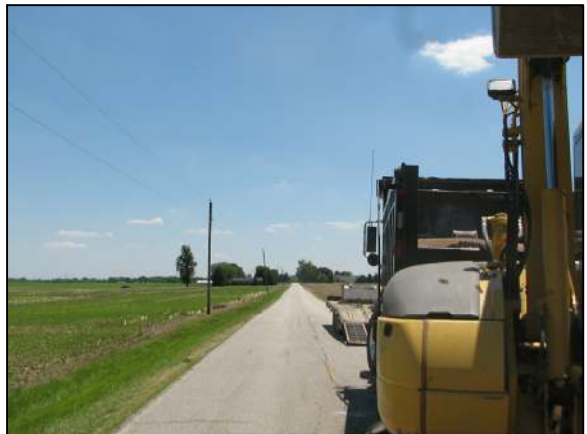
View from above the stone looking south along County Road 150 West (Witt Road.)
