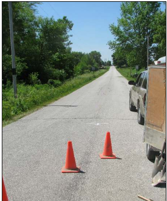
View from above the stone, looking south along County Road 150 West (Witt Road.)
